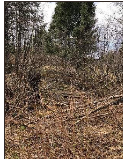
Figure 9: Image decaying bridge over stream crossing on western side of Pananen road
